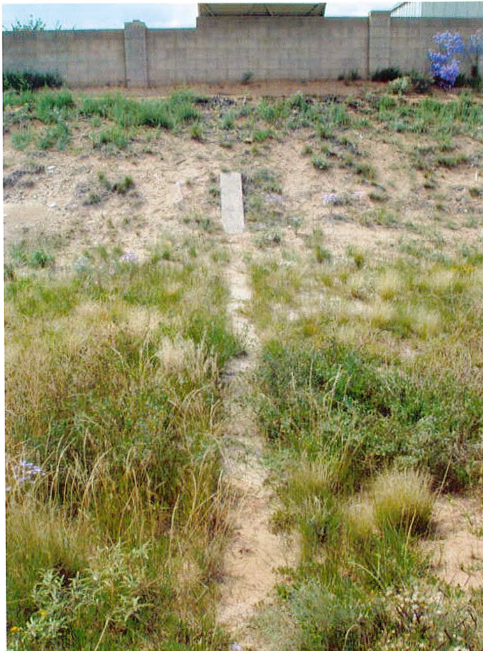
GRADE CONTROL IN EARTHEN CHANNEL SOUTH OF VANCOUVER ROAD
