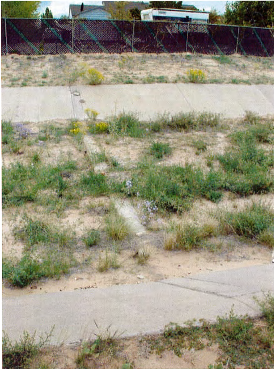
EARTHEN BOTTOM, PAVED SIDE SLOPE CHANNEL WITH GRADE CONTROL NORTH OF PECOS LOOP
