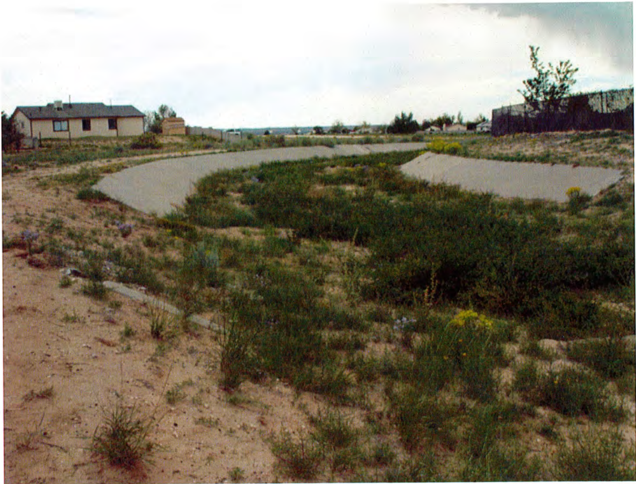
TRANSITION FROM EARTHEN TO PAVED SIDE SLOPE CHANNEL LOOKING SOUTHWESTERLY
