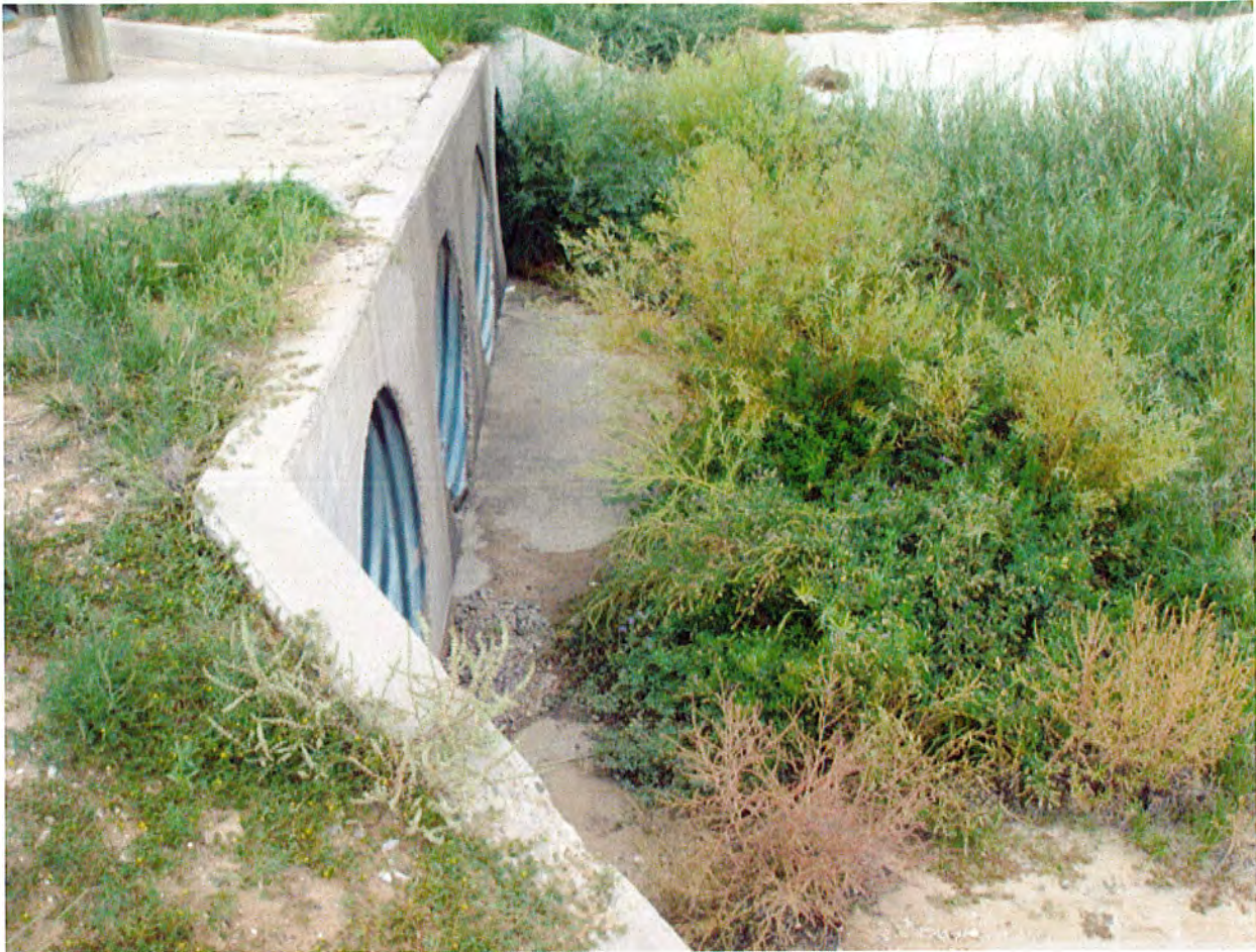
4-48" CULVERT OUTLET AT PECOS LOOP
