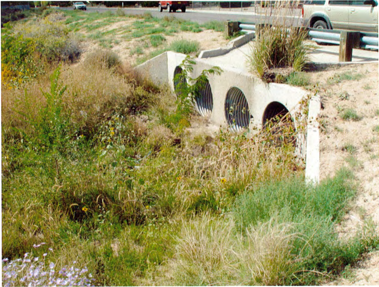
4-48" CULVERT INLET AT PECOS LOOP
