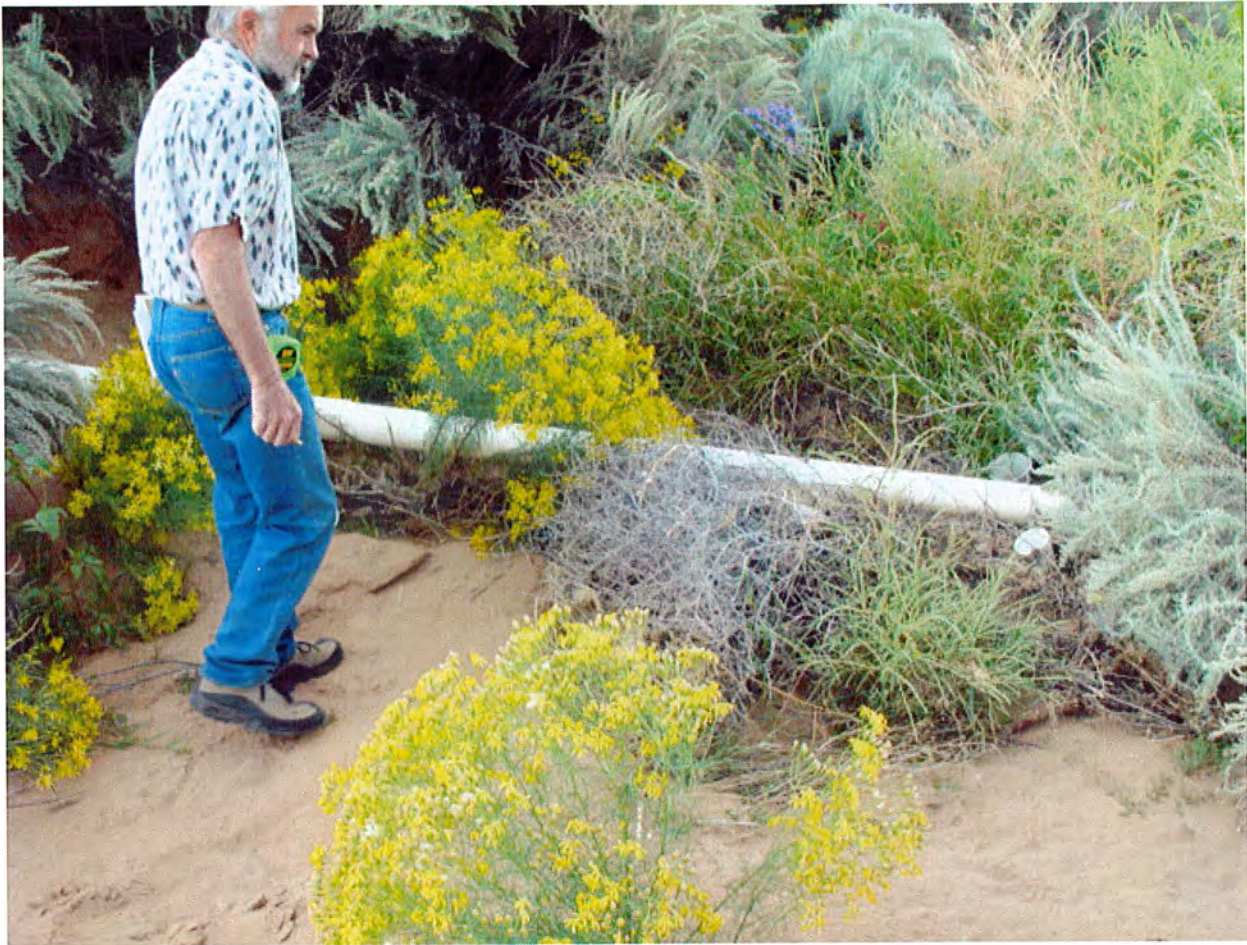
“PARK CHANNEL” EXPOSED UTILITY NORTH OF SOUTHERN BOULEVARD
