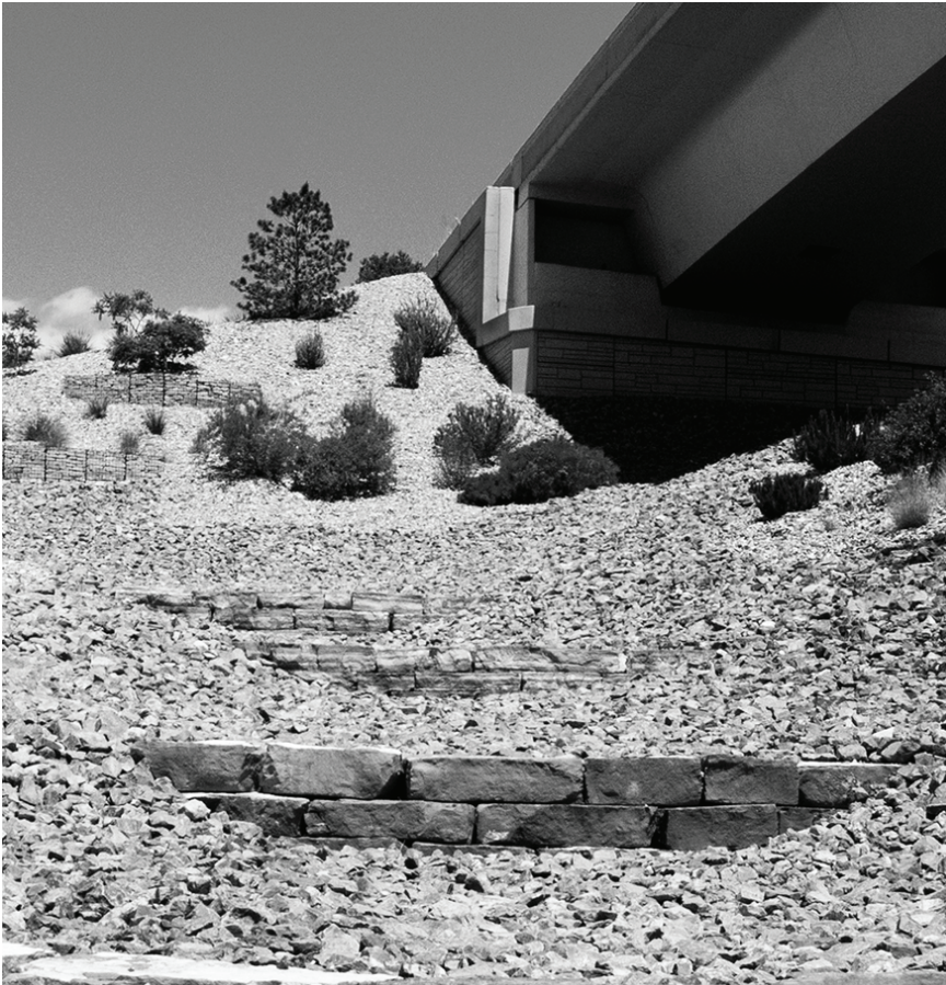
Check dams and gabions slow runoff
