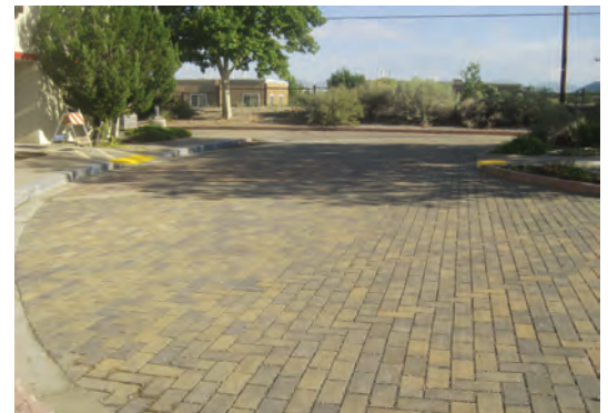
Permeable Pavers At Traffic Circle Entry
