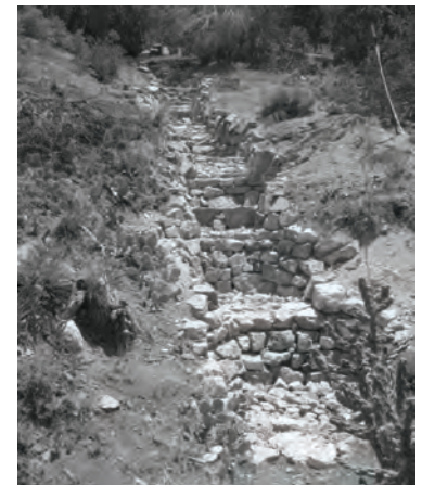
Installation of a rock-lined ditch with step pools, mitigates stormwater flooding.
