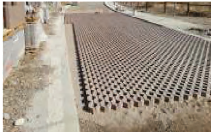
Setting Permeable Pavers On Prepared Subbase
