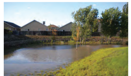
Ponded stormwater spreads into native grass meadow following 1" rainfall
