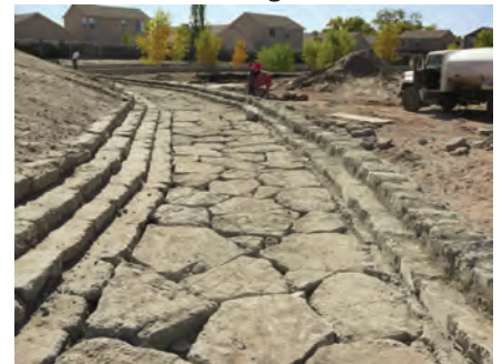
Bioswale lined with recycled concrete sidewalk slabs reused from nearby streetscape project
