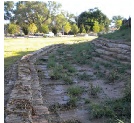
Bioswale lined with recycled concrete sidewalk slabs reused from nearby streetscape project
