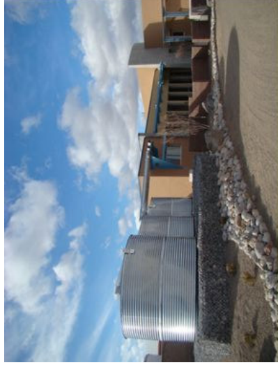
Top left: 4,600 gal. cistern. Top right: Three new cisterns total capacity over 15,000 gal. used for landscape watering.
