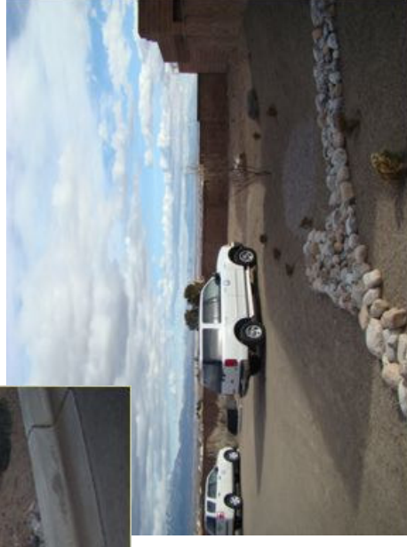
Above: on-site ponding reduces runoff. Right: pervious parking lot and small catch basins for infiltration.
