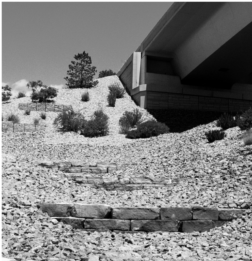
Check dams and gabions slow runoff
