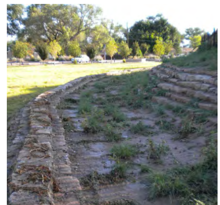
Bioswale lined with recycled concrete sidewalk slabs reused from nearby streetscape project
