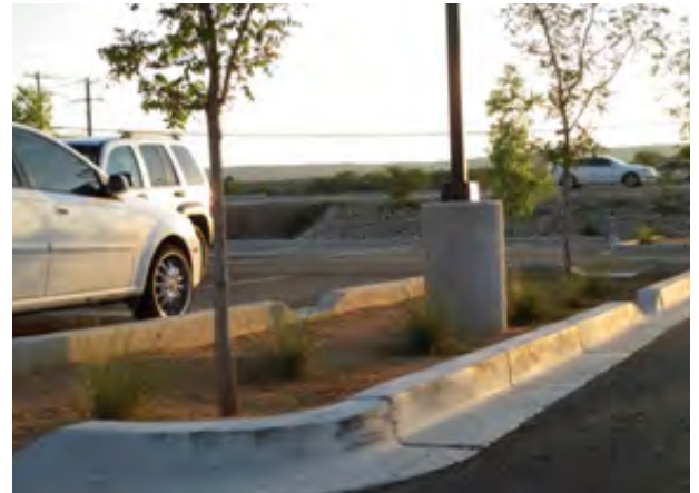
Water harvesting infiltration swale with curb cuts
