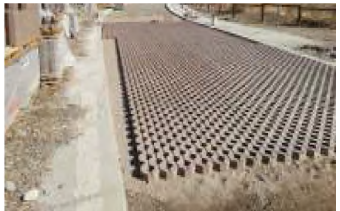
Setting Permeable Pavers On Prepared Subbase
