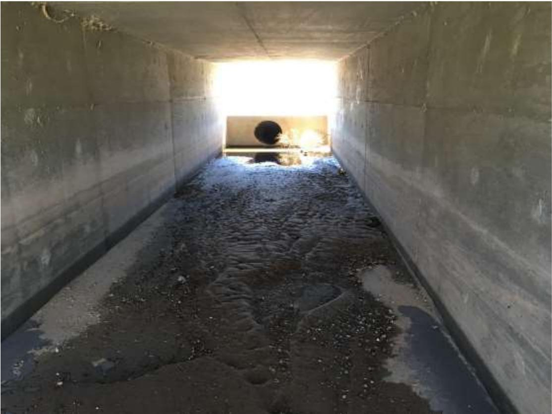
Flows diverted from south barrel of road crossing to water quality meander for treatment. This barrel has a stormdrain inlet from large commercial development west of project site
