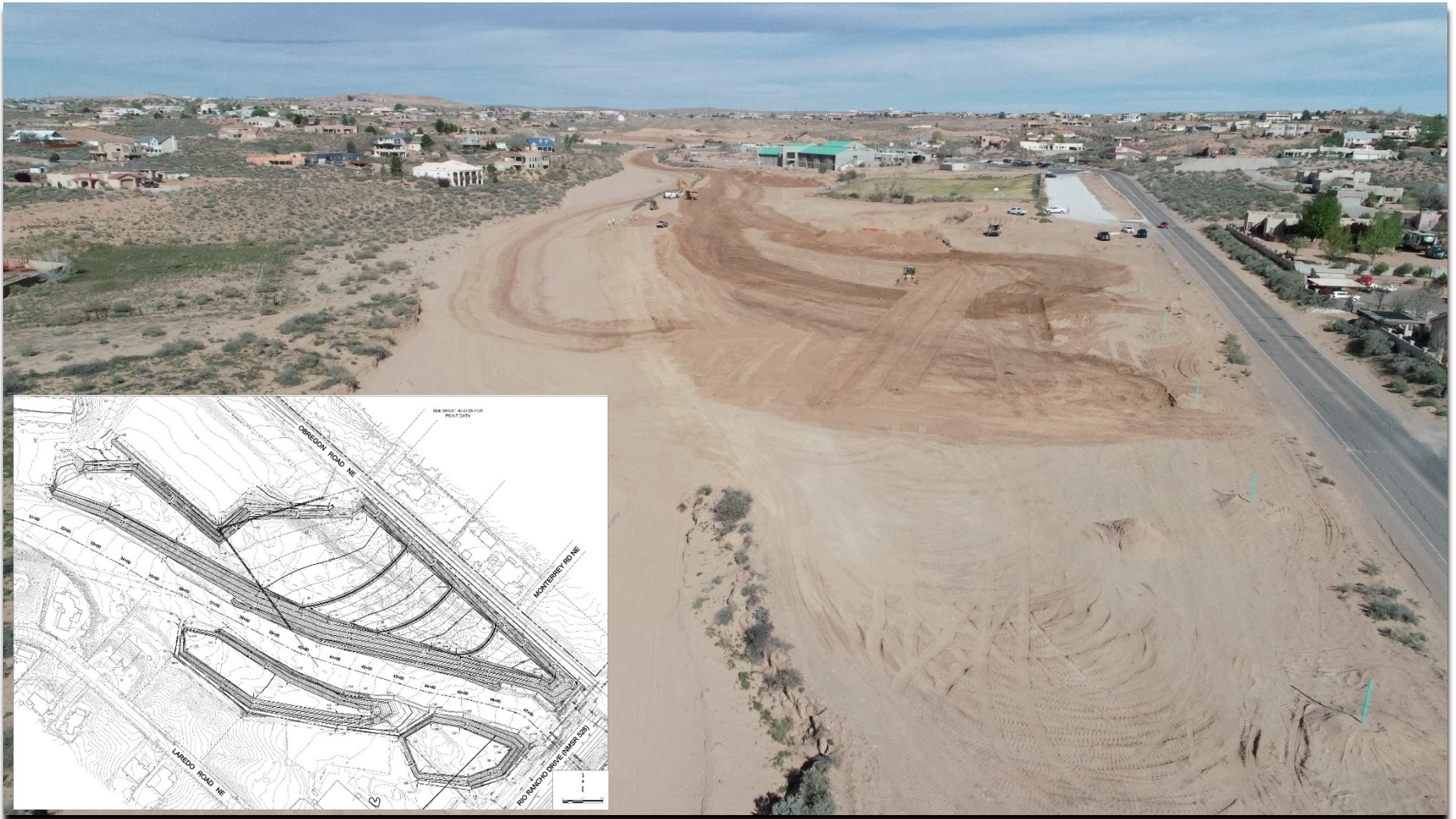
Figure 2 - Sediment disposal and channel stabilization downstream of Saratoga Rd.
