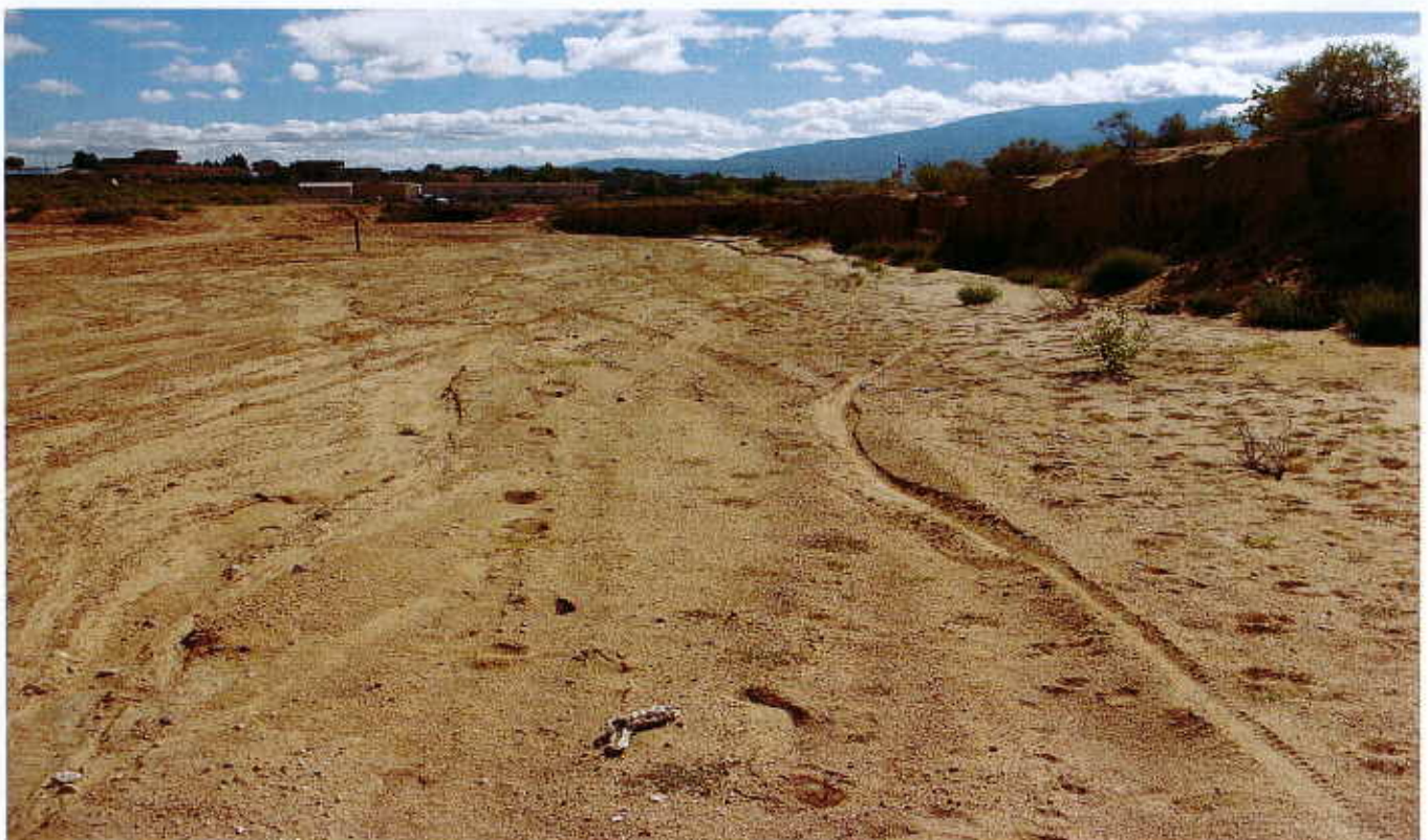
Lomitas Negras Main Branch looking downstream from previous photo at the Saratoga Road and 2 – 6 ft rise x 12 ft span box culverts
