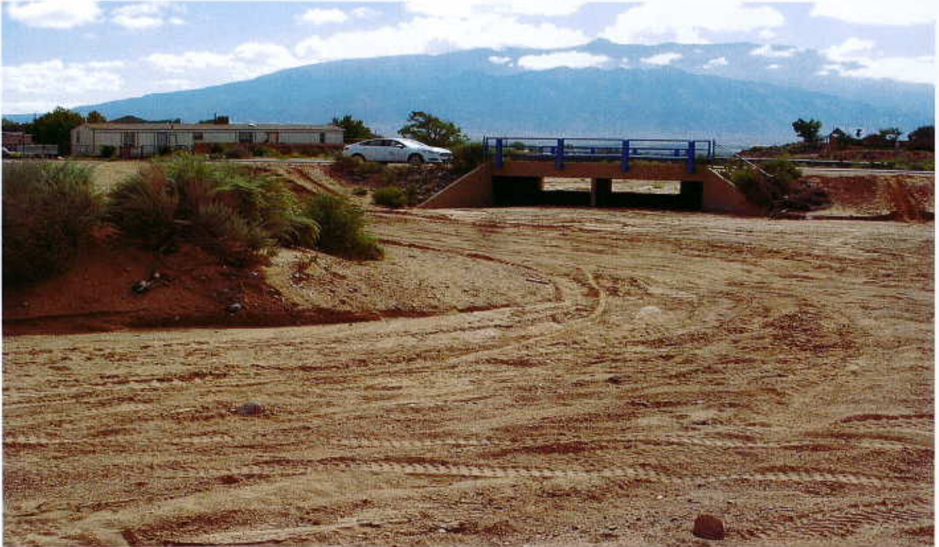
Lomitas Negras Arroyo North Tributary (left) at confluence with Main Branch (right) looking downstream - east at Saratoga Road Box and 2 - 6 ft rise X 12 ft span box culverts
