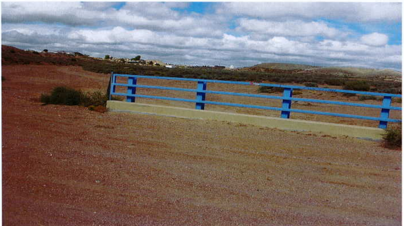
Standing on Saratoga Road looking west at Lomitas Negras Arroyo Main Branch on left and the North Tributary on right at location of red marker on blue rail. Location of the proposed Saratoga Pond.
