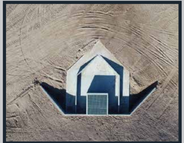
Overhead view of water quality tower at Lomitas Negras facility
