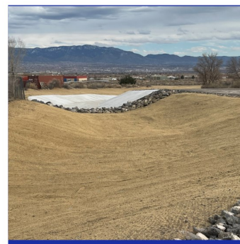
Ivory Channel Bank Stabilization Project
