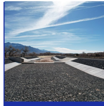
Lower Venada Bank Stabilization Project
