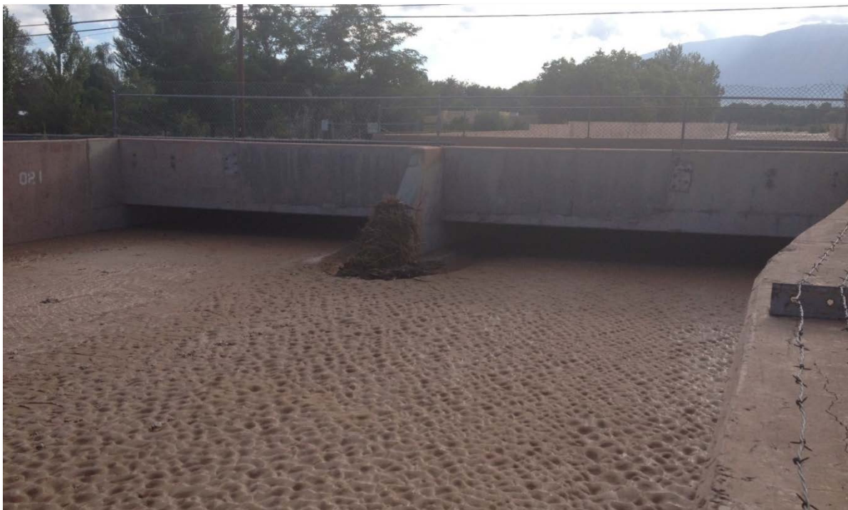
Figure 3.4: Flow (top) and sediment accumulation (bottom) in the Harvey Jones channel caused by storms in September 2013 (image source: SSCAFCA archive).
