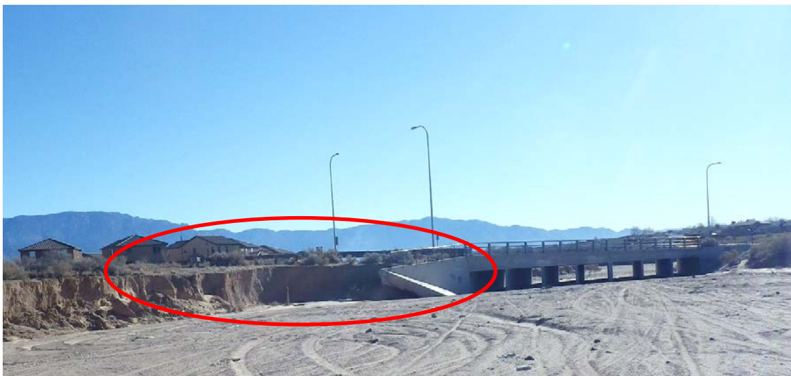
Figure 3.17: Erosion at the left bank wingwall of the crossing structure at Broadmoor Blvd.
