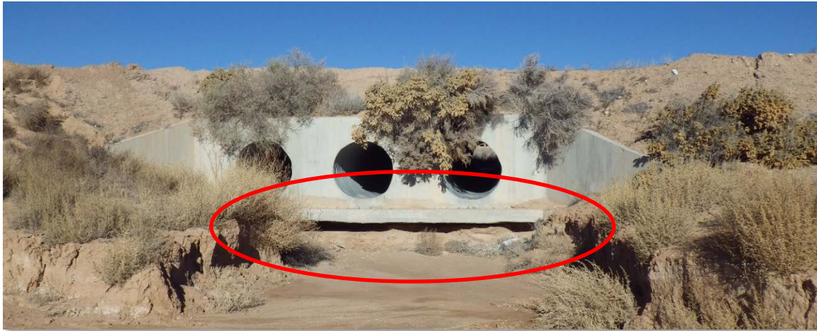
Figure 3.16 Degradation downstream of a crossing structure at Idalia Rd. on the Lomitas Negras tributary.
