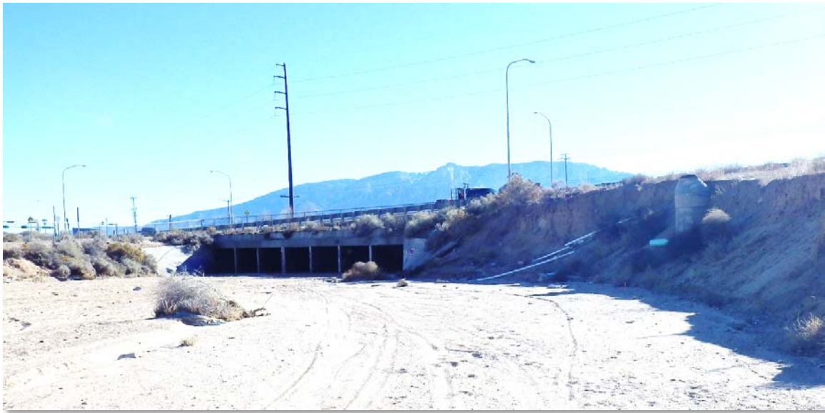
Figure 3.18: Erosion at the right bank wingwall of the crossing structure at New Mexico 528.
