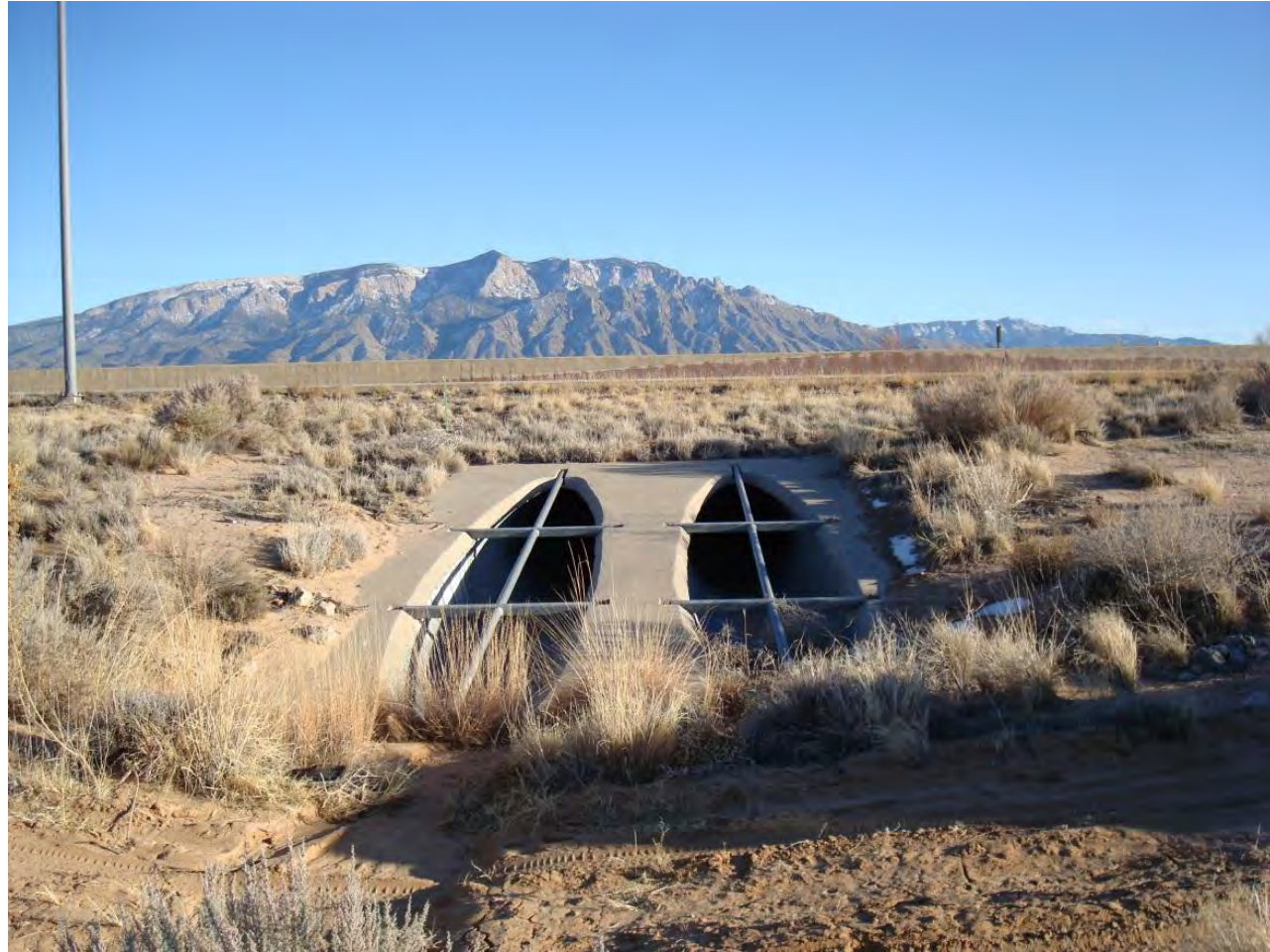
Photo 13: Culverts at NM 528 and Basin A (2 –60” CMP, capacity \approx 335 cfs)
