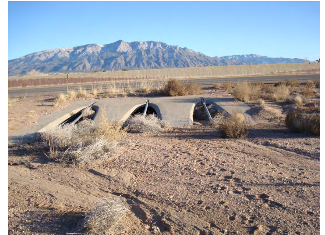
Photo 15: Crossing WC_04X (3 – 60” CMP, capacity ≈ 422 cfs)
