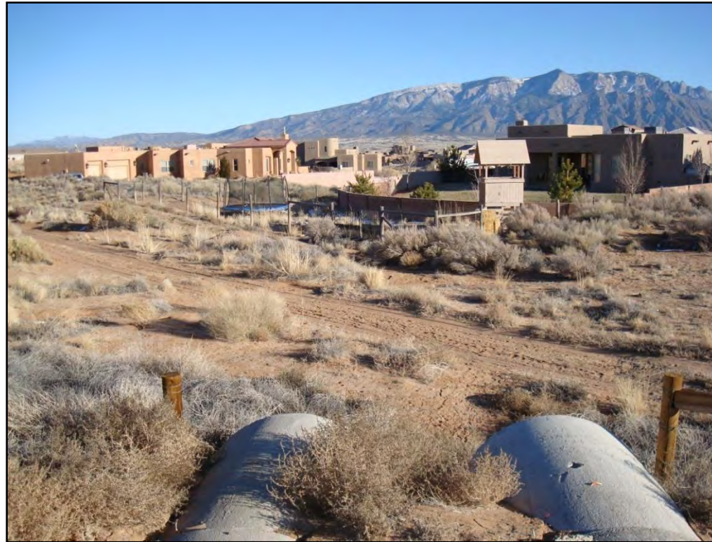
Photo 9: Home located in former flow path of Arroyo, looking east from SAD 6 Pond # 6; the outlet structure of the pond (two reinforced concrete pipes) can be seen at the bottom of the photo.
