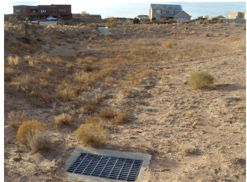
Photo 6: Christopher Pointe Pond (WC_06P, capacity \approx 2 AF), with outlet structure in the foreground.
