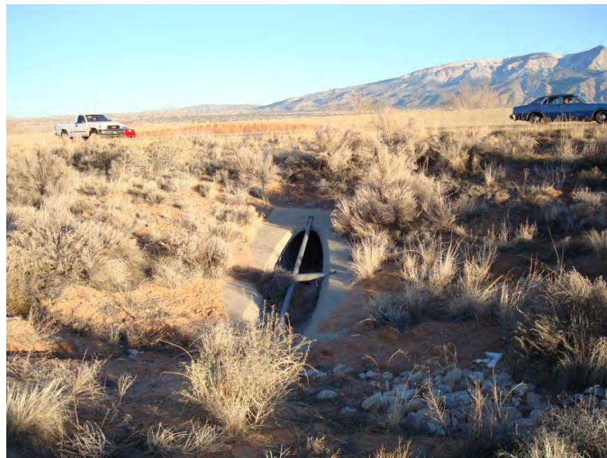
Photo 16: Crossing WC_05X (left, 1 – 36” CMP, capacity ≈ 46 cfs) and WC_06X (right, 1 – 36” CMP, capacity ≈ 71 cfs)
