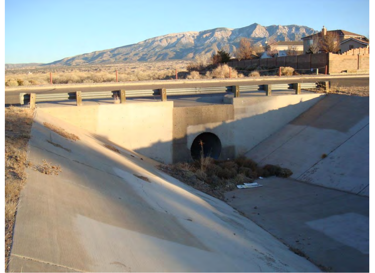
Photo 14: Culvert at Willow Creek Road and Basin A (1 –66” CMP, capacity \approx 290 cfs)
