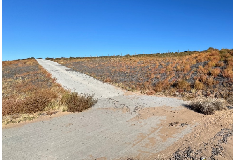
Figure 3 Reinforced concrete ramp and apron configuration.
